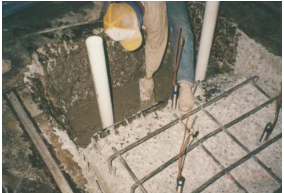
14. ...and the grout poured into the large excavation. The surface of the concrete had earlier been primed with epoxy resins.
