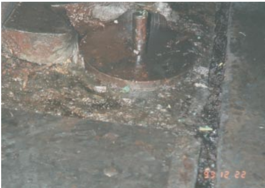
3. The channel on the right hand side of the photo is the top of the vibration damping expansion joint..
