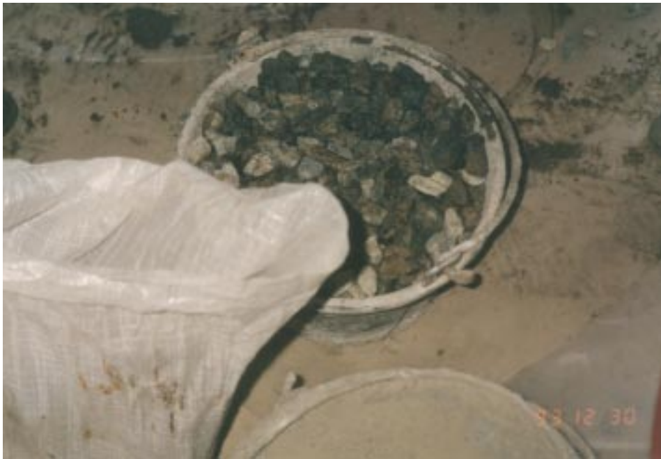
13. ...crushed stone aggregate added...
