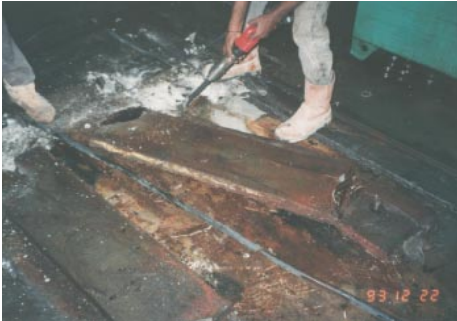
5. The bond between the existing soleplates and the grout was very poor..
