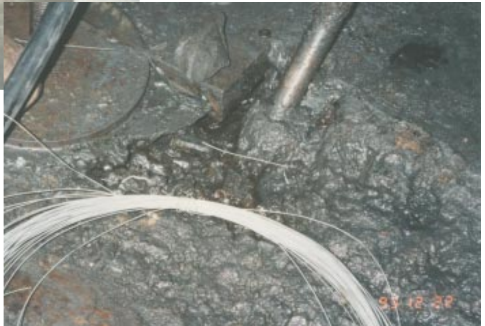
3. The channel on the right hand side of the photo is the top of the vibration damping expansion joint..
