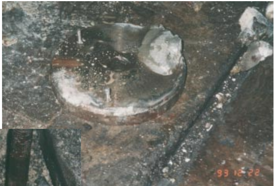
5. The bond between the existing soleplates and the grout was very poor..
