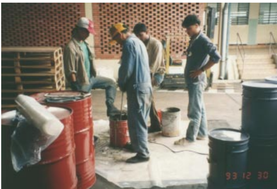
12. cement grout was mixed....
