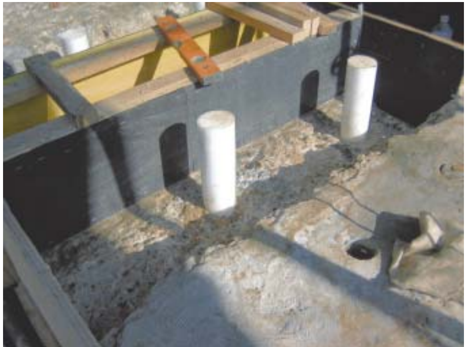
18. 17 July 2005. ALPHATEC 800 epoxy grout poured to give a working level for installation of the soleplates.
