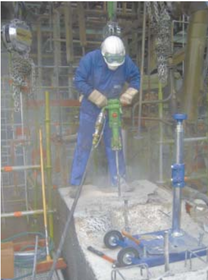
14. Cores were drilled to 1000 mm from the foundation surface to ensure full removal of the existing bolts.
