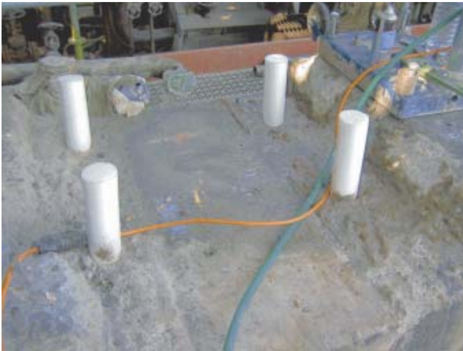
17. Formwork set in place, with a polypropylene liner stapled to the inside of the plywood as a release barrier.
