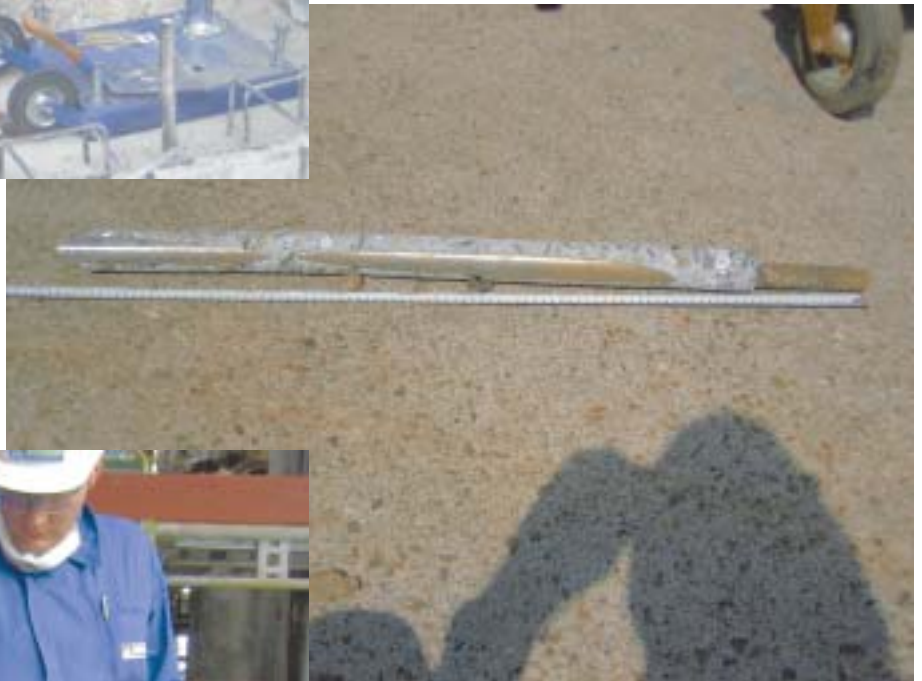
15. Diamond core drilling is a tedious business that continued throughout the week, in order to complete the removal of 10 anchor bolts.
