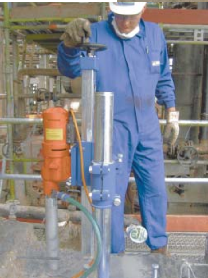
14. Cores were drilled to 1000 mm from the foundation surface to ensure full removal of the existing bolts.
