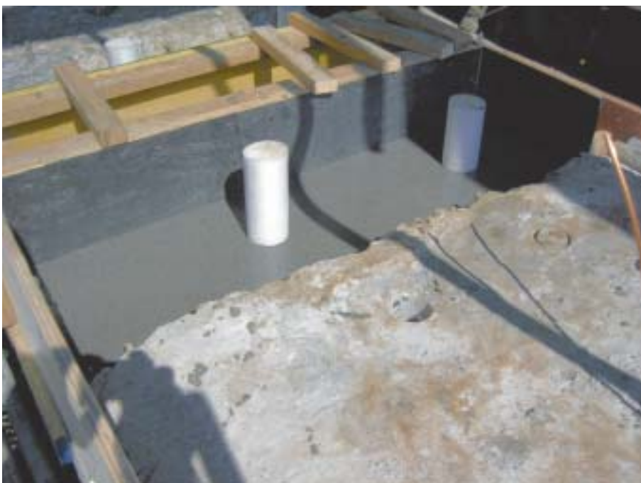
18. 17 July 2005. ALPHATEC 800 epoxy grout poured to give a working level for installation of the soleplates.
